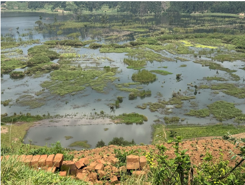
Water Retention Facility (non-functioning), Kisoro District, January 2025
