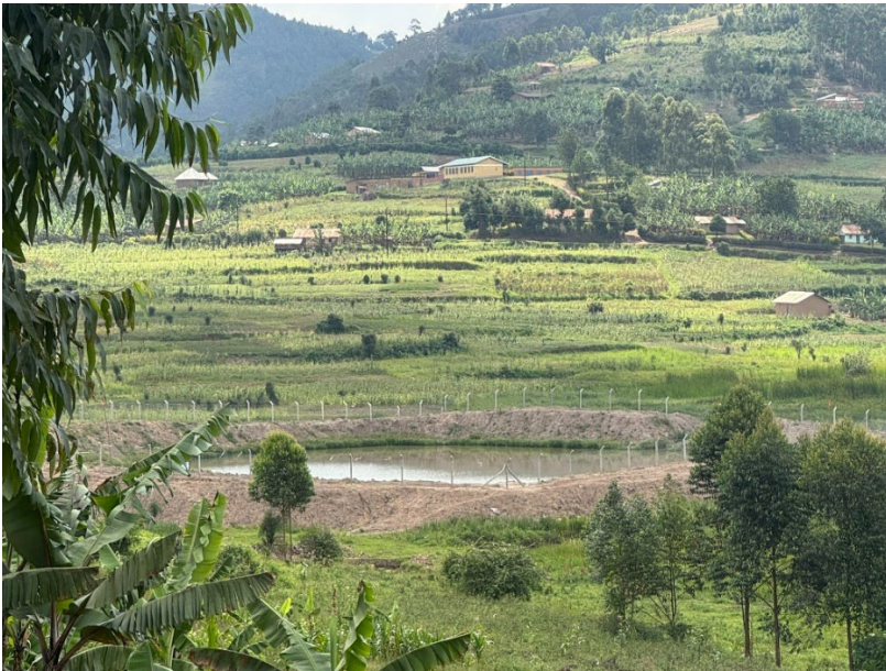
Water Retention Facility, Rukiga District, January 2025
